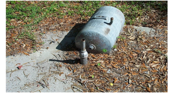
Abandoned wells offer a ready path for contamination and must be properly plugged.
