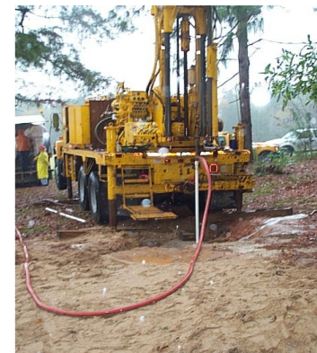
Drill rig set up on site.
